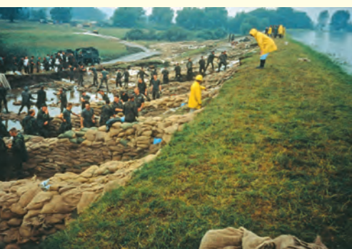
Fortifying a dyke along the Oder River during a flood, 1997
