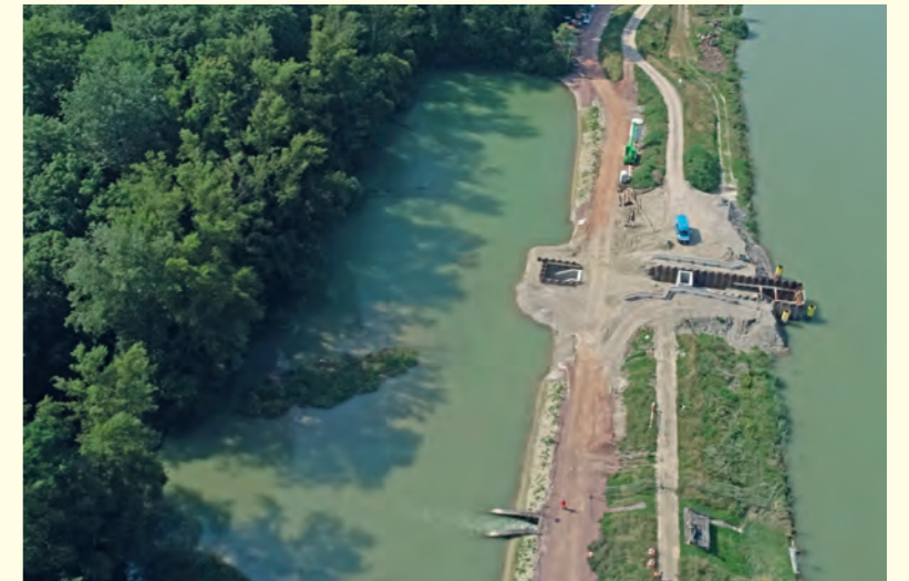
Construction site of an inlet structure in the Breisach/Burkheim retention area
