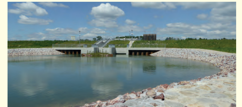
Inlet structure at the Elzmündung retention area
