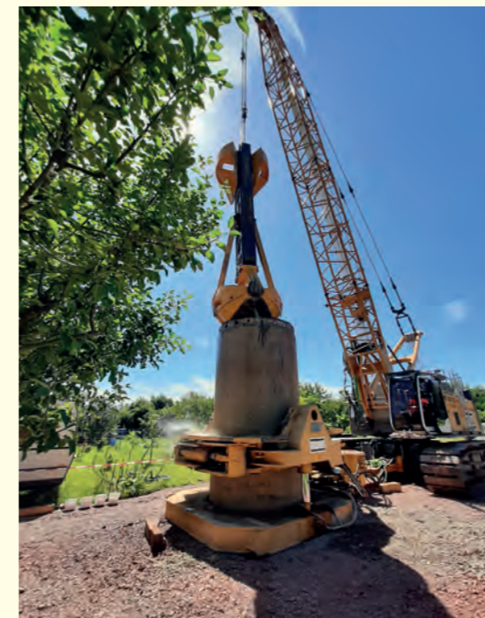
Drilling a well
