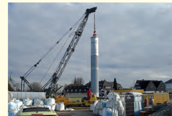
Installing a well pipe in a well shaft
