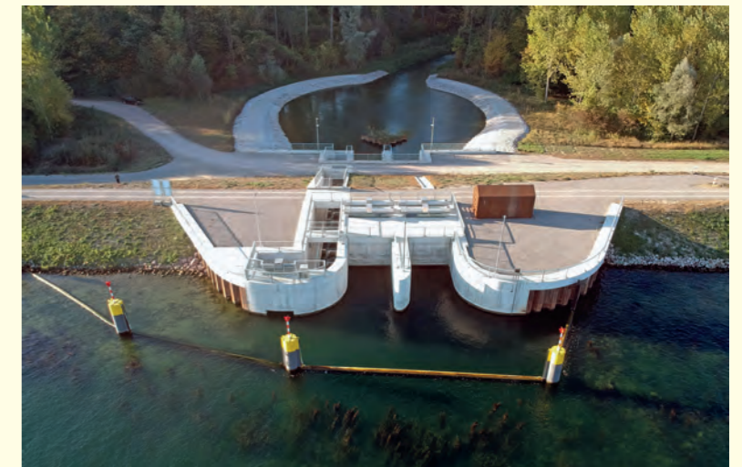
Central inlet structure at the Elzmündung retention area
