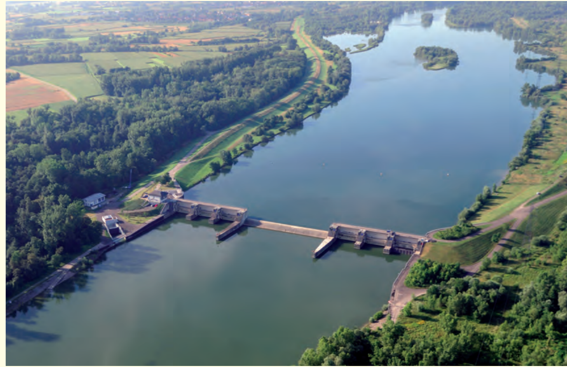
Aerial view of the retention area near the Kehl/Strasbourg irrigation barrage
