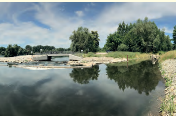
Inlet structure of the Elzmündung retention area
